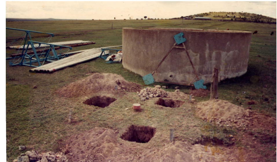
Foundation holes dug, prior to placing the jig over them to locate the Foundation Bolts. The tower jig can be seen in the back ground.
