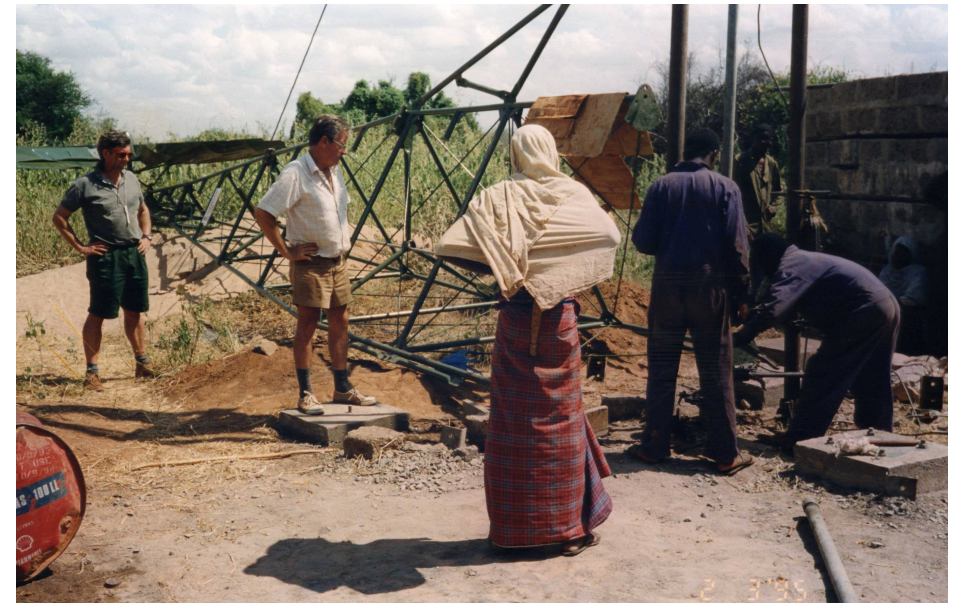
Foreman Paul Muiruri winches the last pipe down, before raising this 16ft Kijito up on its hinged tower
