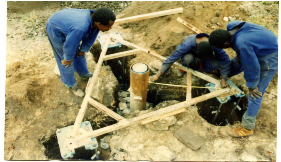
The Foundation jig with the tower footplates and the foundation bolts attached. As can be seen it is important to adjust the jig so it is centrally located around the borehole casing
